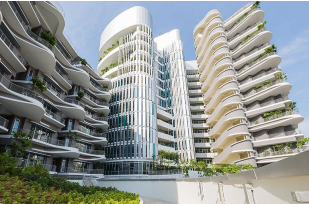
Ng Teng Fong Hospital in Singapore (Studio 505, HOK, CPG Eng) Natural Cooling 70% patient rooms, each bed with garden
